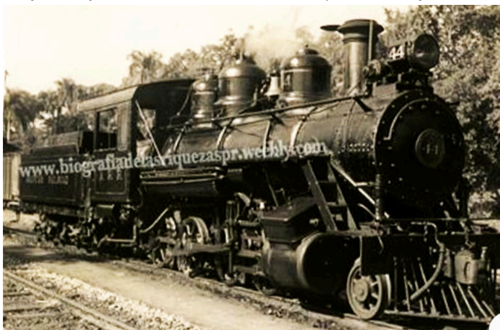
Note the much higher running plate, possibly after rebuilding with a superheated boiler.
