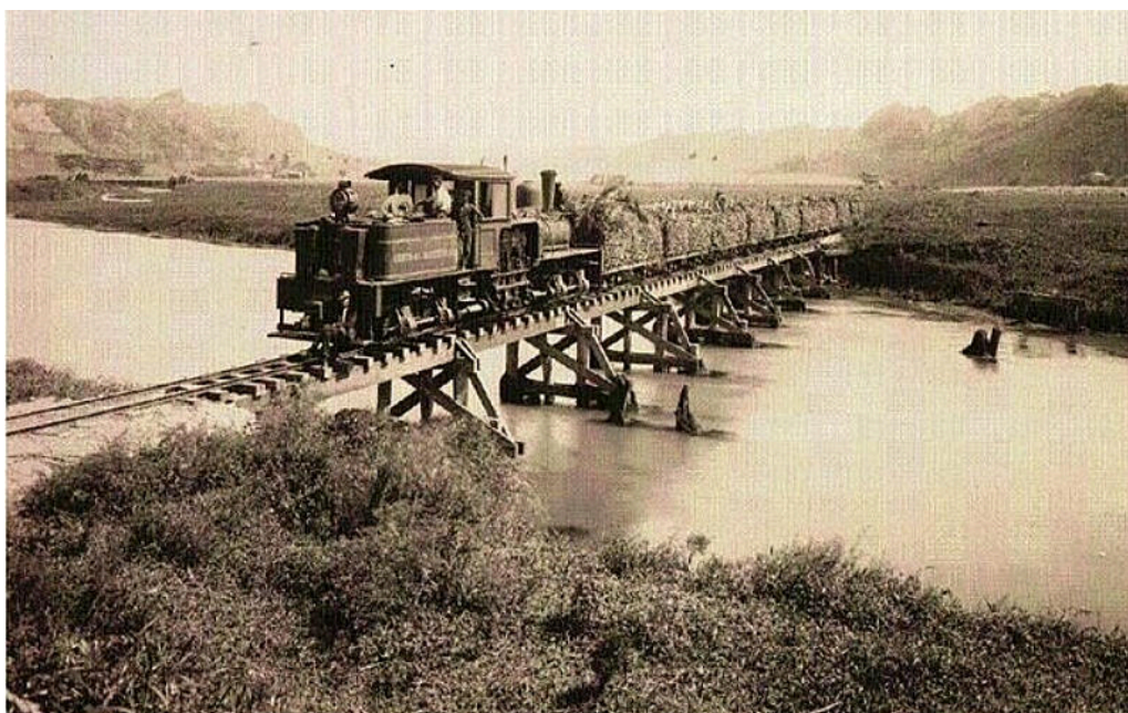
One of Central Monserrate's 60cm gauge Shays hauls a loaded cane train to the mill, date unknown.
