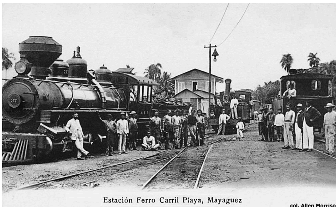
A pair of Cail 2-6-0Ts in the yard at Mayaguez, along with a very different beast, one of the four Baldwin Mallets.
