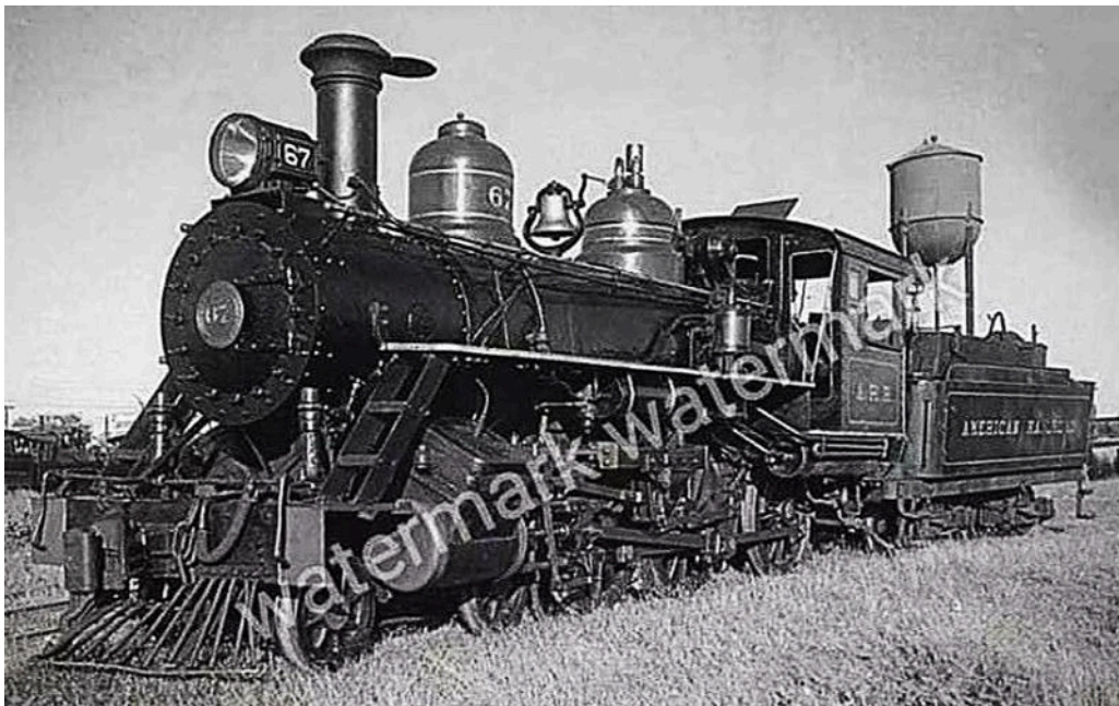
Compound no. 67 shows off its large low pressure cylinder.
