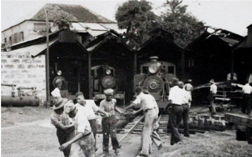
Bridgetown roundhouse during the 2' 6" gauge era. The loco being pulled onto the turntable is one of the 2-8-2Ts, whilst further to the left are the two smaller Baldwin tank engines.
