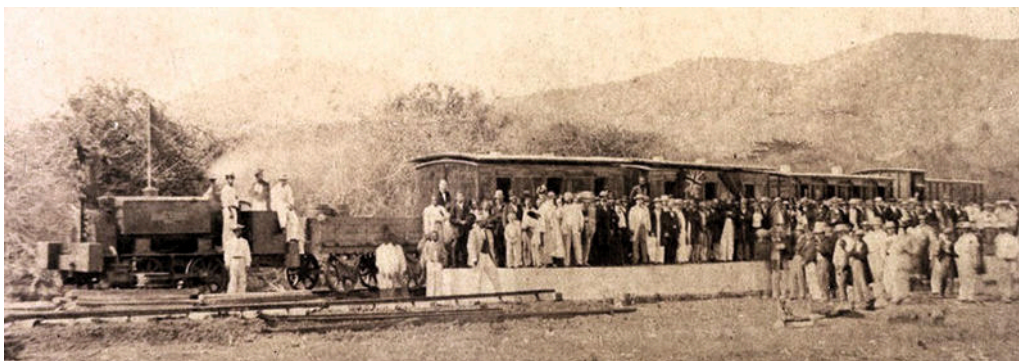
The only known photo of the Central Railway, possibly taken during the opening ceremony for the first stretch, or maybe showing off the construction works.
