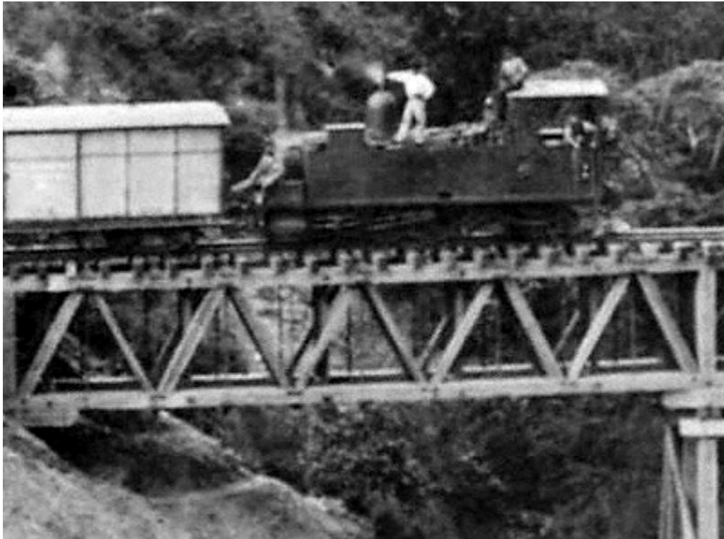
One of the first batch Nasmyth-built 0-6-4Ts on a timber truss viaduct. As usual the loco is running bunker first. Date unknown.
