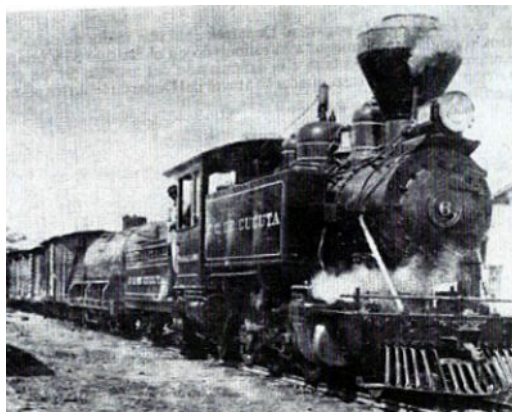
The same design of 2-6-2T was to be seen later posing as no. 6 on the FC de Cúcuta , with added tender and a different spark arresting stack.
