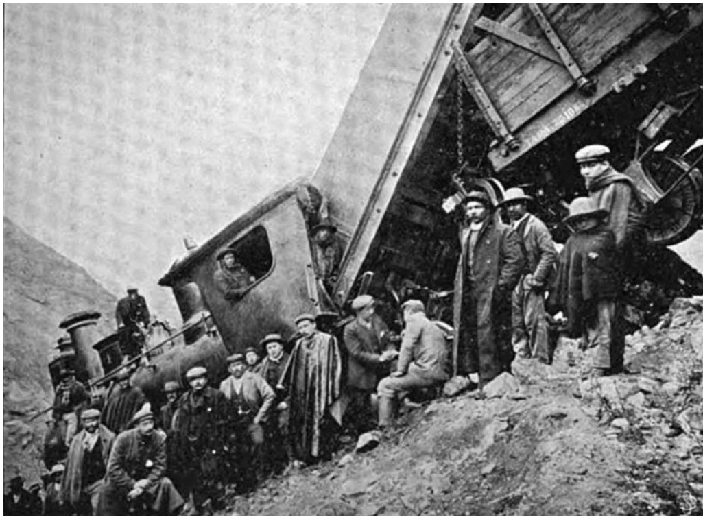
One of these NBL 2-8-0s appears to have met with an accident. Details unknown. Rather strangely, the engine seems to have a rectangular boiler-mounted sandbox, rather than the original saddle style or the dome on the previous page.
