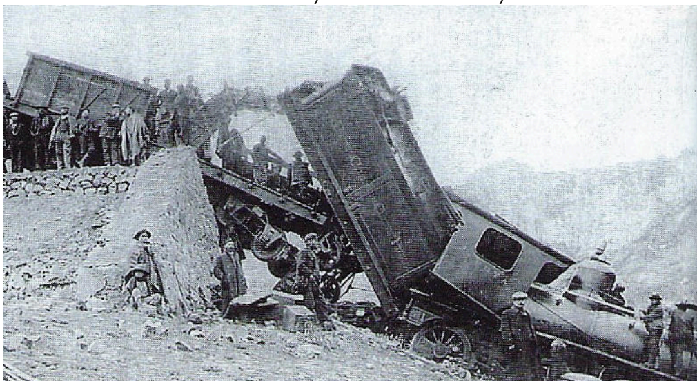
No 1 'OROYA' after a derailment. Note the later cab and boiler. Photo apparently from Ian Button collection as reproduced in the late Bob Whetham's book [5] vol.2.
