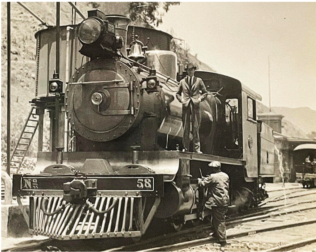
No. 58 after rebuilding.
