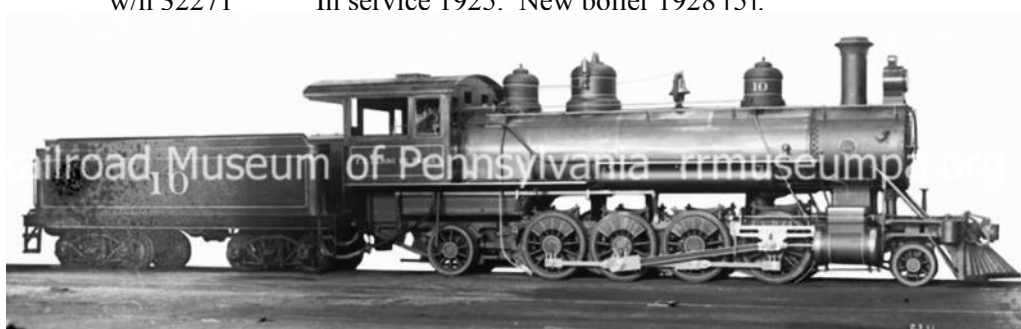
This image is from Baldwin negative 02311 and hi-res copies can be purchased from the Railroad Museum of Pennsylvania. Note that this engine carries slide valves, unlike all the later photos of these machines which show piston valves.
