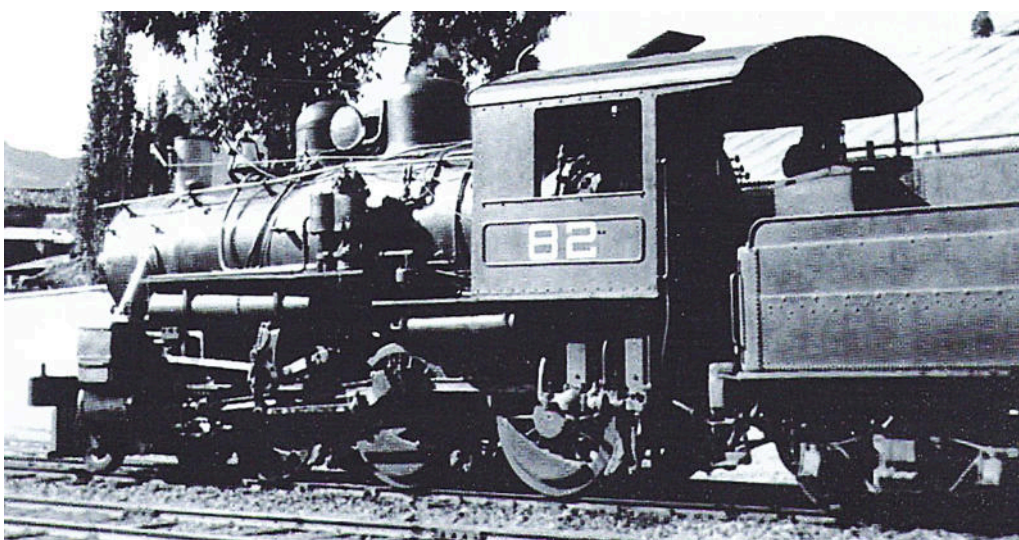
No. 82 again, this time at Ayaviri, and with an additional mysterious device between sand dome and steam dome. It cannot be the turbo-generator, for the exhaust pipe from that is still visible just ahead of the cab, as it was in the previous photo.
