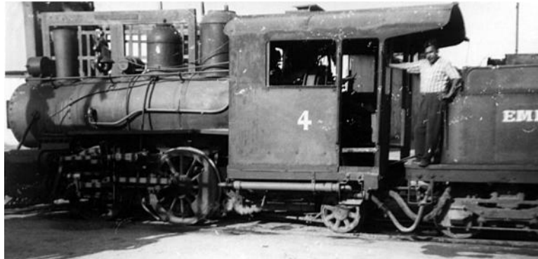
A pair of photos of Eten no. 4 , by courtesy of Garth Samuel and Richard Pelham. The cab with its rounded roof eaves may well have originated in the 1955 rebuild. It is interesting that the locations of the domes remained constant throughout the loco's life.
