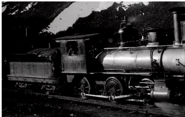
This image bears the loco name ' CALLAO ', suggesting that it was these earlier Rogers moguls that carried the big rectangular sandboxes rather than the more common sand-domes.
