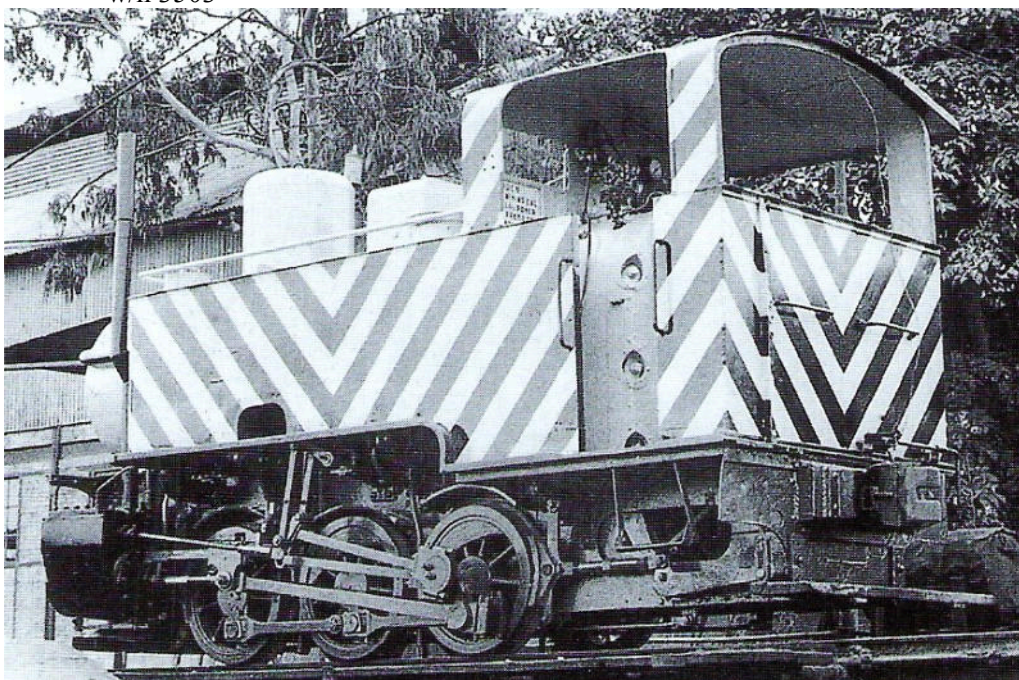
Loco converted to fireless, probably originally one of this pair of O&Ks.
