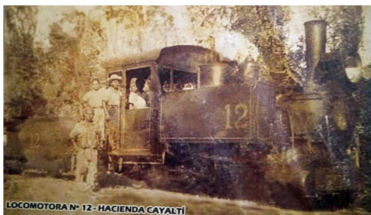
Loco no. 12 , ex International Petroleum Co. Photo courtesy of Sr. Julio Gamboa.
