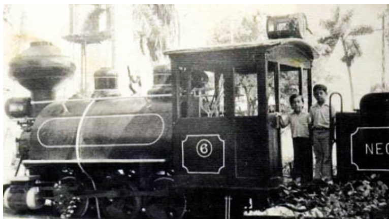
Hacienda Tumán no. 6 , seemingly retro-fitted with a Rushton stack, and possibly with a name beginning 'NEG...' on the tender.
