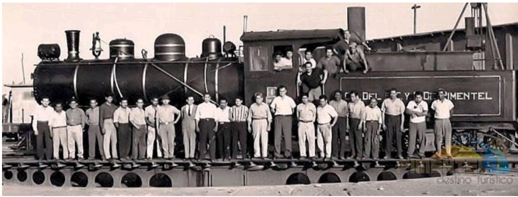
This photo, taken on the turntable at Pimentel, shows no. 1 after it had regained the front sand-dome. There also appears to be an oil-fuel tank on the tender.
