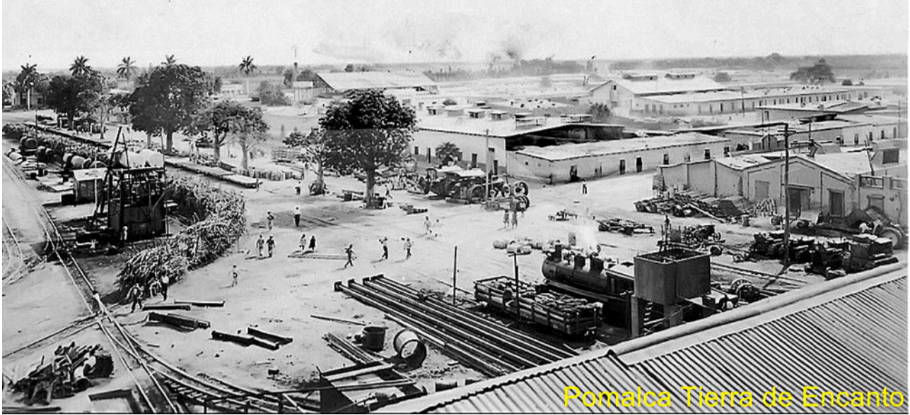
An overview of a yard at Hacienda Pomalca, with a large tender loco to the right and also steam traction or maybe ploughing engines also visible. -----
