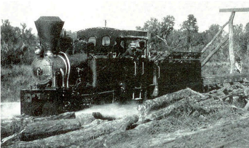
Interestingly, this engine appears to have squarish spectacles as seen on no. 7 at Puerto Casado though the cab is rather different. It may be the same engine though with the cab later having been rebuilt using the original spectacles.
