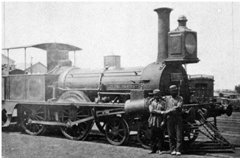
This photo of the Argentine FC Oeste loco no. 19 'LUZ del DESIERTO', also built by Sharp Stewart though some years later, shows the characteristic horizontal valves driven by push rods above inclined cylinders.
