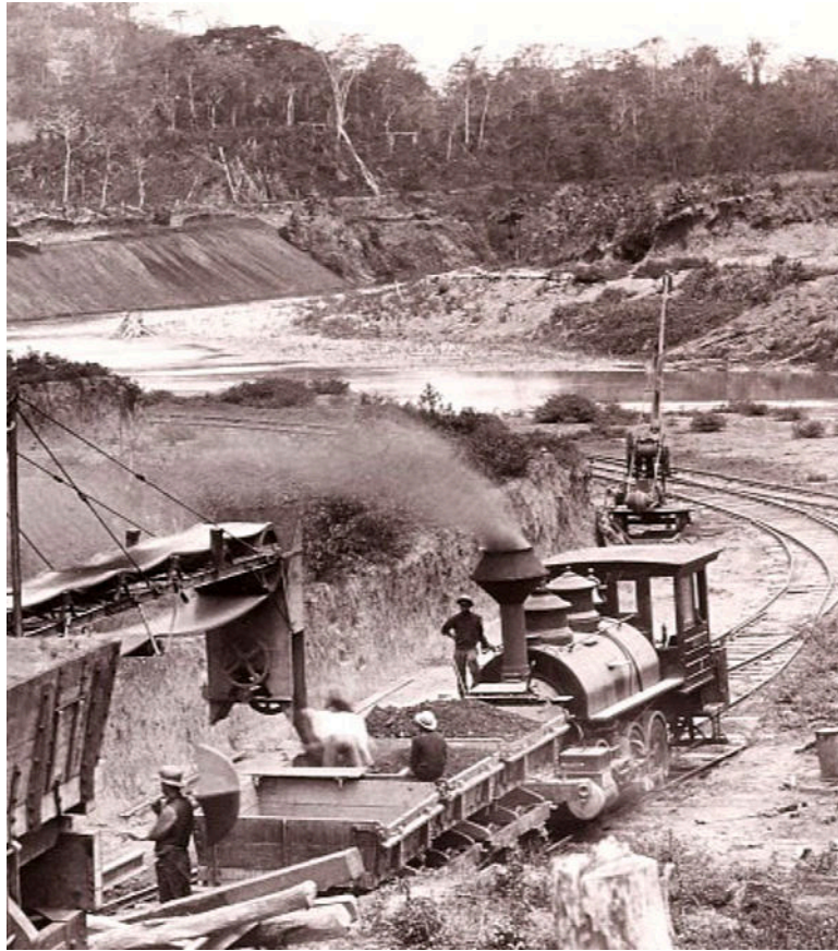
A Rogers 0-6-OST on a construction or excavation site. The year is unknown but the conveyor belt to the left suggests a relatively late date, ie. during the US era rather than the French one.
