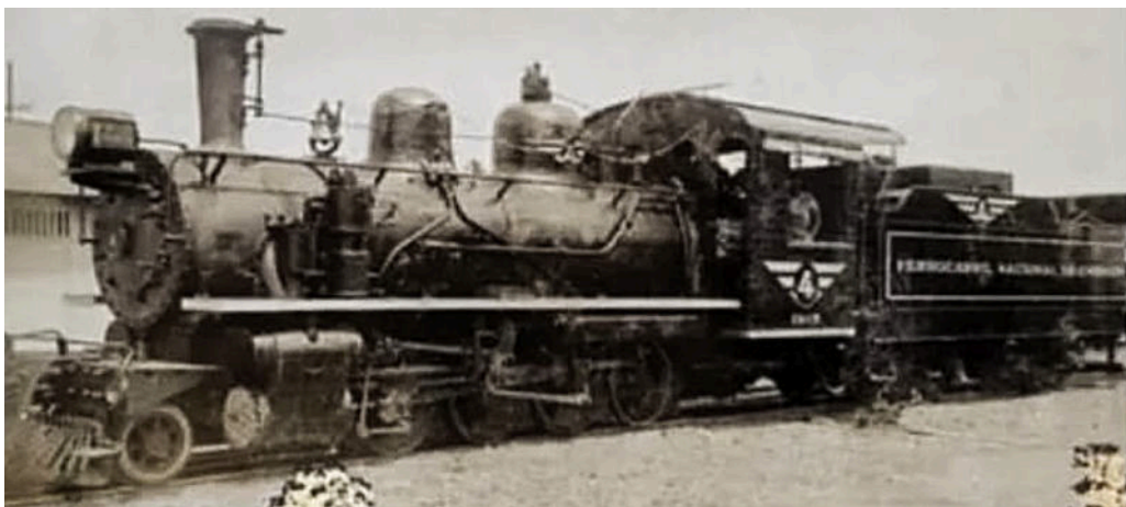
No. 4 was clearly an updated ALCo version of no. 3 , with piston valves instead of slide valves and almost certainly oil-fired.
