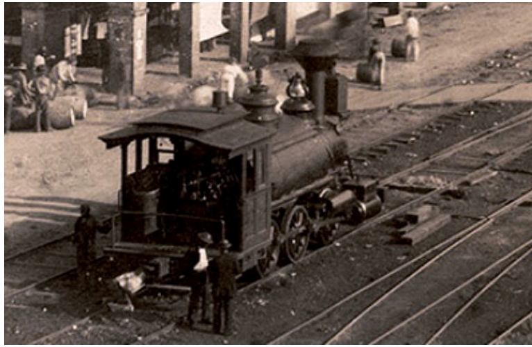
A Hinkley 0-6-0ST standing in Colón (Aspinwall) station prior to 1885. It rather looks as though the rear wall of the cab has vanished to leave just fresh air and a single low handrail.
