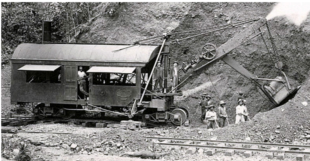
A steam excavator in use during construction of the G&QR. No technical details are known.
