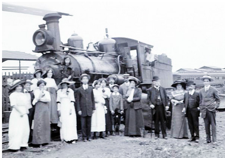
Two views of 4-6-0 no. 6 , identifiable by its dome over the firebox, a feature which distinguishes it from all the later G&Q locomotives.
