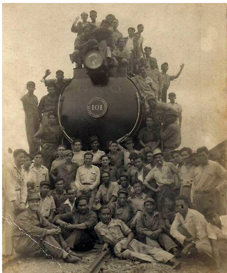
Two unattributed photos provided by courtesy of the late Gavin Hamilton show how the Garratts were rebuilt with cylindrical tank and bunker aligned to the boiler in Algerian style. 'FERROCARRILES ECUATORIANOS' is painted along the vertical plates at the top of the tank, and 'G. & Q.' across the circular front. It also would appear that this engine has a round-topped firebox, and it may therefore have been no. 101 after its explosion in 1933.
