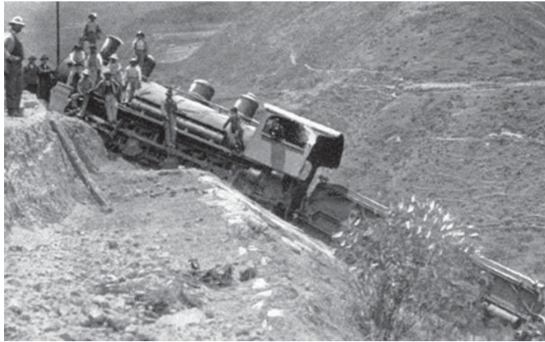
An accident to one of the Vaucrain-cylindred locos, as shown in the Baldwin Magazine during the 1920s. This image may well have been reversed for publication, unless the air reservoir on one or more of these engines had been moved to the right hand side. However, it has been reversed again here.
