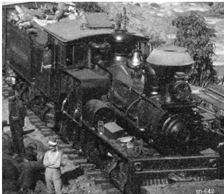
This photo of no. 16 from the Shay website at https://www.shaylocomotives.com/ shows only one minor difference from no. 15 above, the much smaller toolbox on the running plate in front of the air reservoir.
