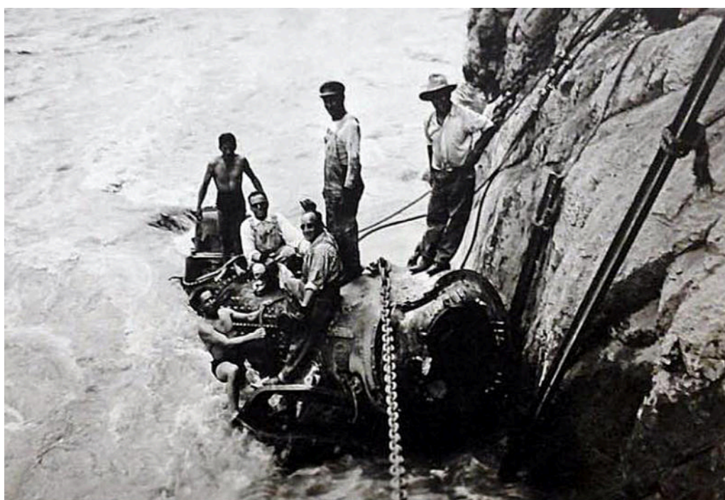
Workers attempt the salvage of a Baldwin boiler from the rushing waters after a wreck.
