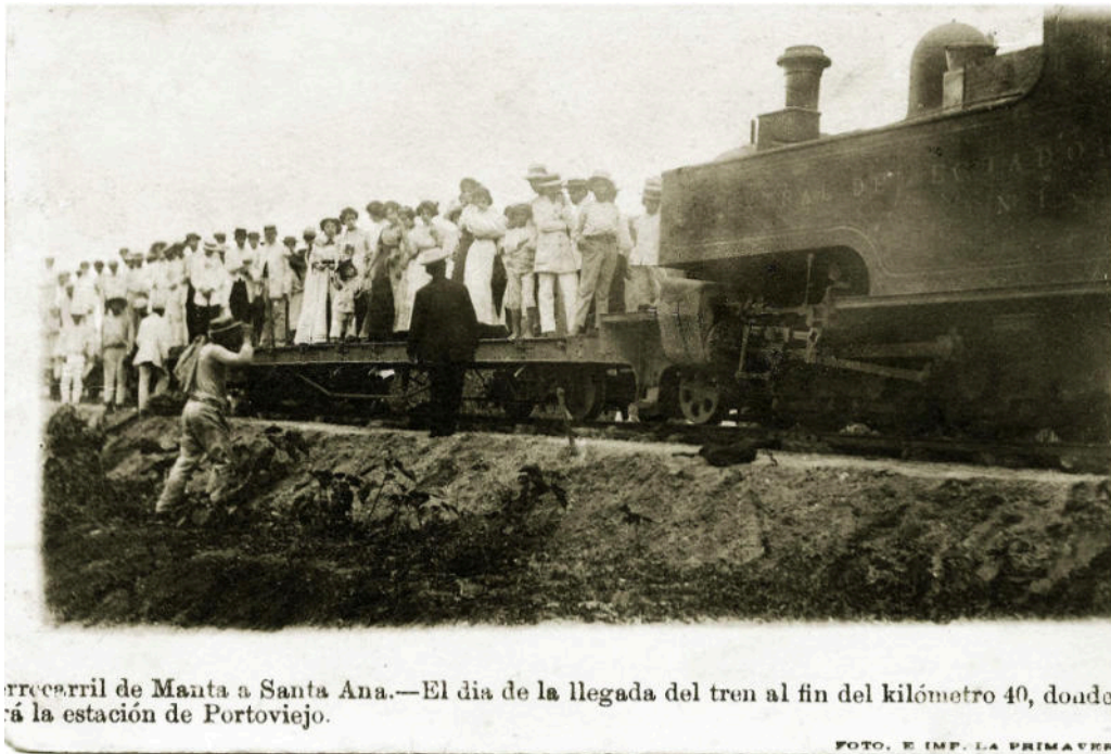
One of the 2-6-2Ts of the FC Central del Ecuador is seen with the first train to reach the site of Portoviejo station. The loco bears the number 1, which conflicts with information gained from other sources.
