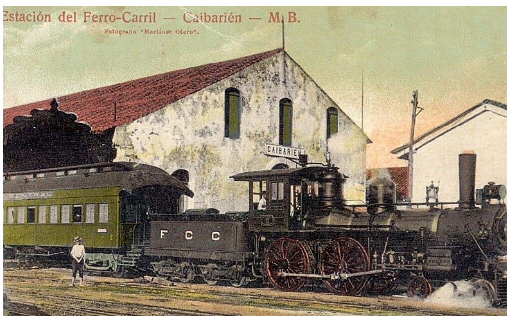
An ancient 4-4-0 at Caibarien, probably inherited from one of the FC Central's predecessors but not yet identified. It carries Rogers plates on the steam-chests and the running number 2 .
