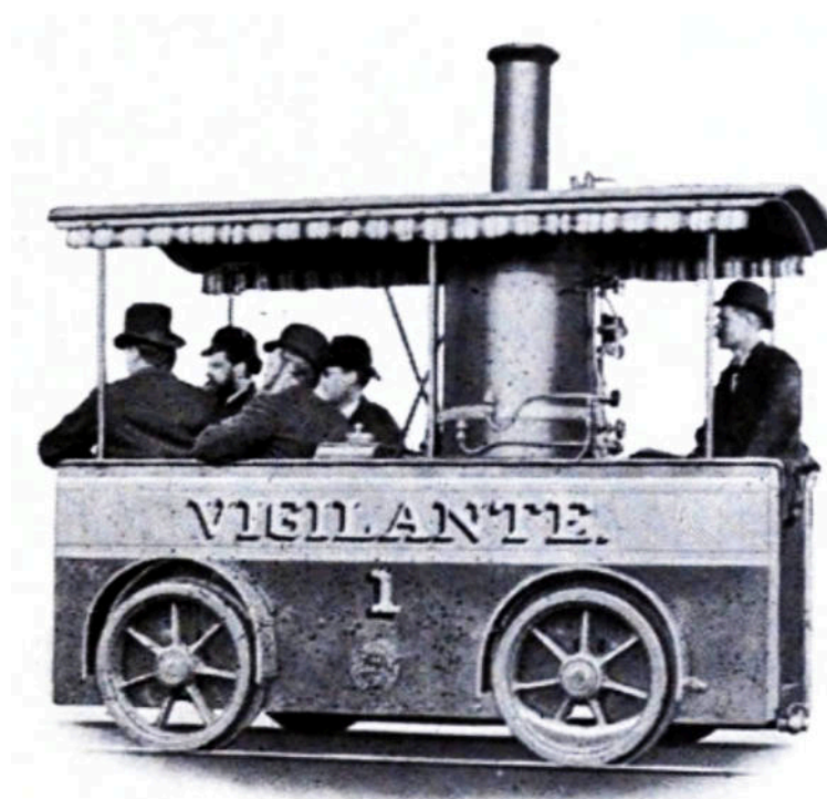
STEAM INSPECTION CAR
