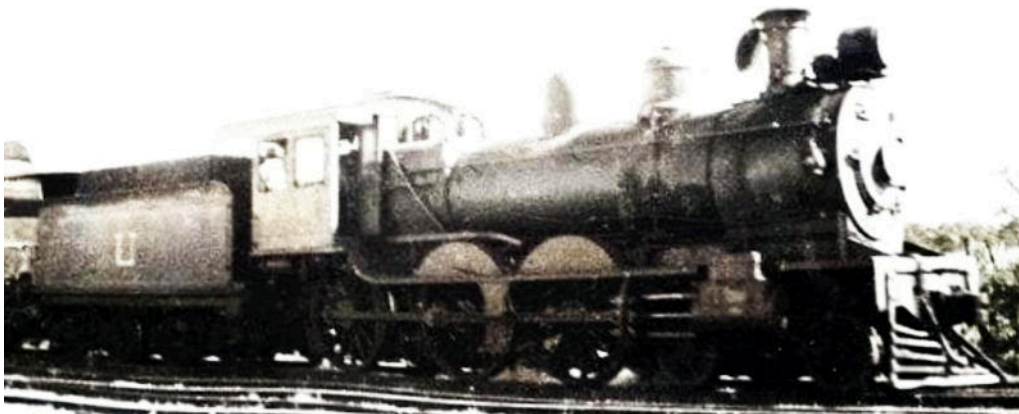
Note the strange up-sloped running plate in front of the cab. Might be a later iteration of the previous photo, after conversion to oil.
