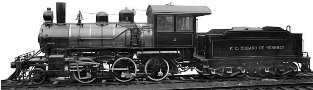
Two photos of no. 2 , the first of the pair of VIW 2-6-0s originally ordered for Serbia, but not delivered owing to the progress of the First World War.
