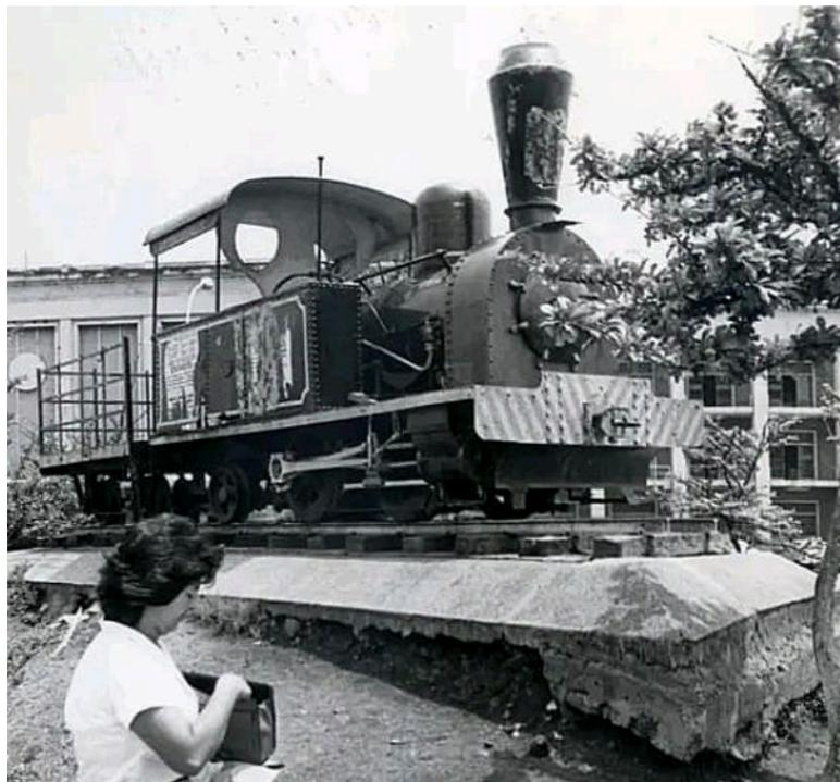
It is clear that the engine as originally plinthed retained its tanks, but these were later lost, possibly as a result of corrosion of the platingwork.
