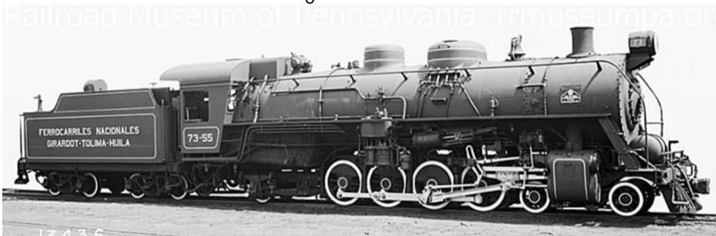
FCGTH no. **73**. Right hand side. Ahead of the two-stage air pump the air-operated reverser can be seen. Hi-res copies of this photo are available from the Railroad Museum of Pennsylvania - BLW negative 13436.
