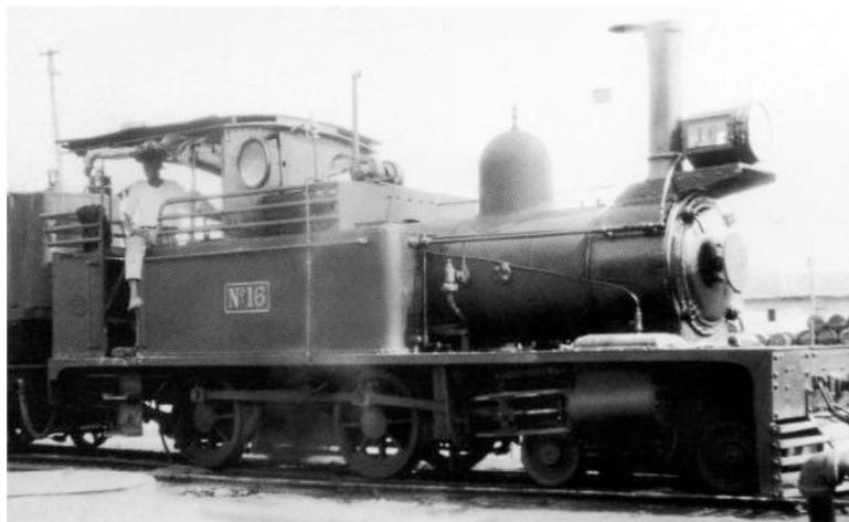
No. **16** as running in 1926 with altered cab, oil tank and added turbo-generator. Photo by P. C. Dewhurst [8].
