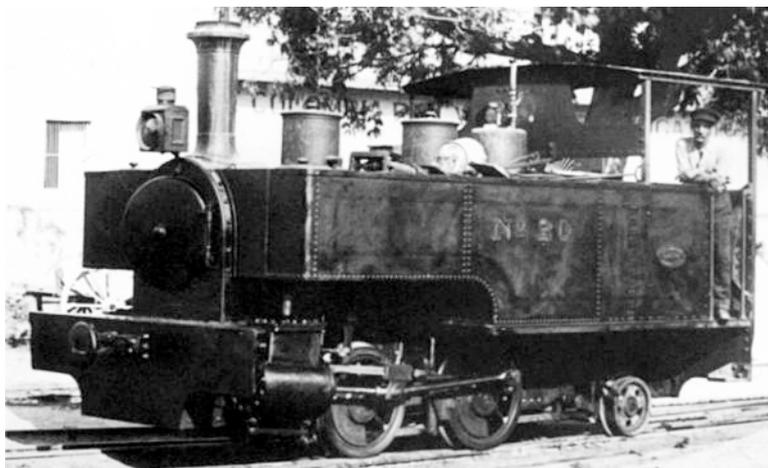
This being no. **20**, it looks as though the 'modified' status of this loco mentioned above consisted of it having side tanks instead of a saddle tank. [8]
