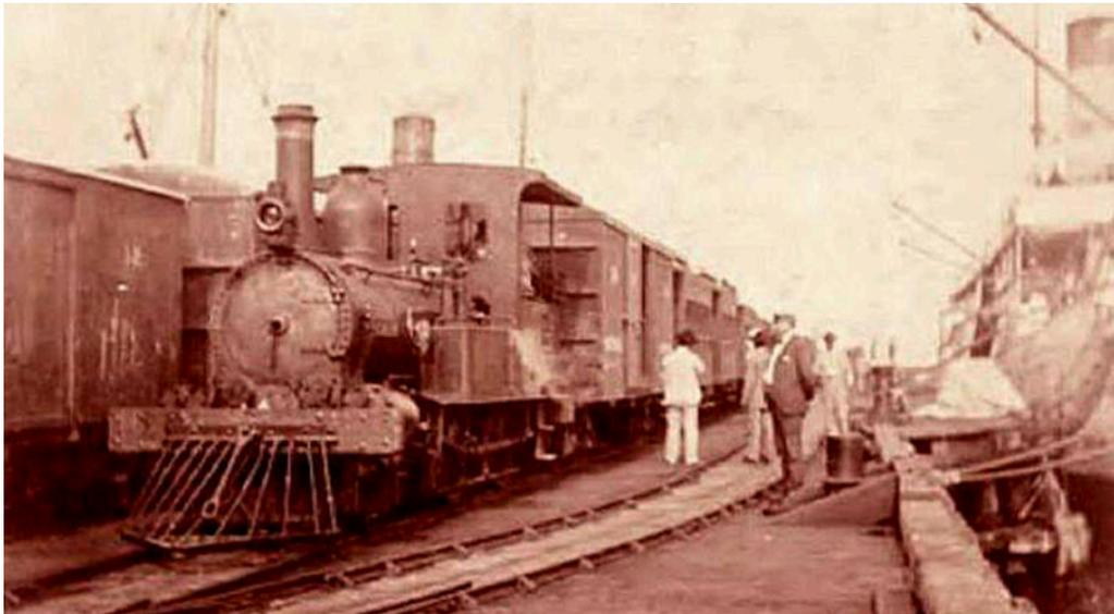
Another view of a Beyer Peacock 2-4-0, this time supposedly at Puerto Colombia in 1903. As well as having had its spark-arresting stack replaced by a straight one, the loco has gained a replacement cab spectacle plate with rectangular rather than round spectacles.
