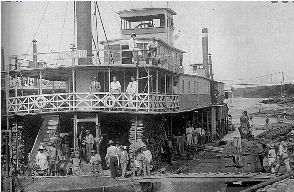
The boiler visible lower right in this view of the stern-wheel steamer 'ADELAIDA' at Girardot, was reputedly the first loco boiler for the new *FC del Nordeste*, and was thus presumably for the Black Hawthorn 0-6-0T 'COLOMBIA' detailed below.
