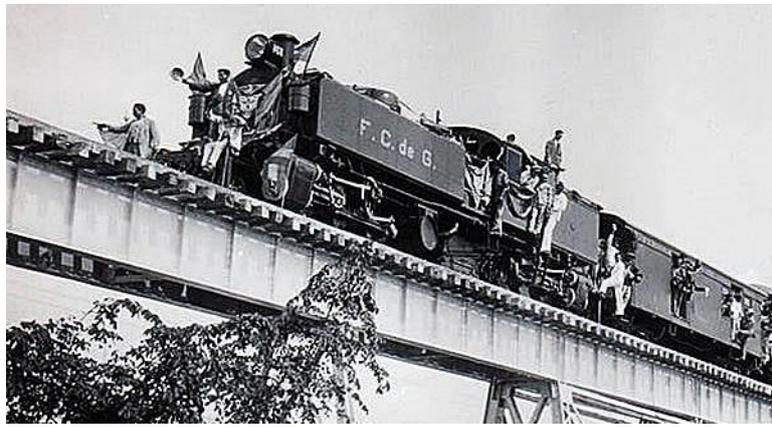
No. **24** at a guess, owing to it having the raised cab roof seen above, and seemingly crossing the big bridge over the río Magdalena. The loco is carrying the drum-shaped sandboxes ahead of the tanks that can be seen in the previous image, but unlike in that photo it retains its capped chimney. The original larger photo was dated January 1<sup>st</sup> 1930, and might even show an opening day train as the bridge was only opened that year.
