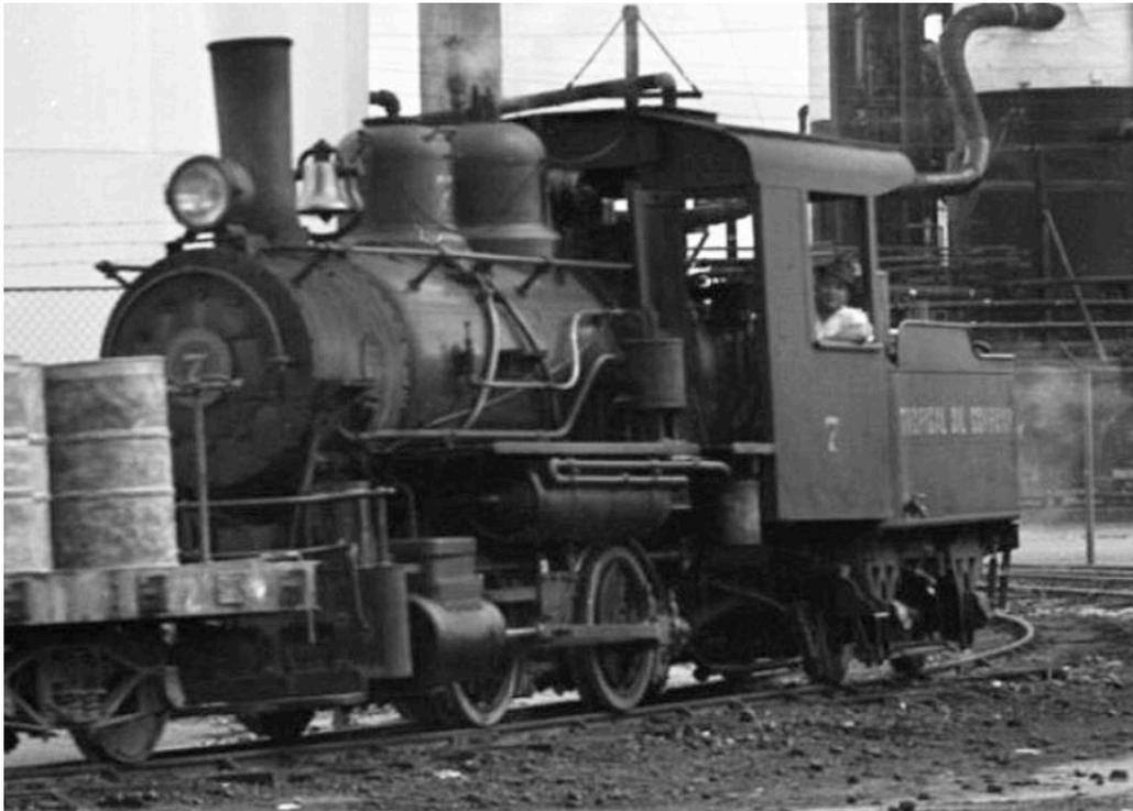
Seemingly the same locomotive, no. 7, but the cab has been replated and has lost the smaller of the side windows.
