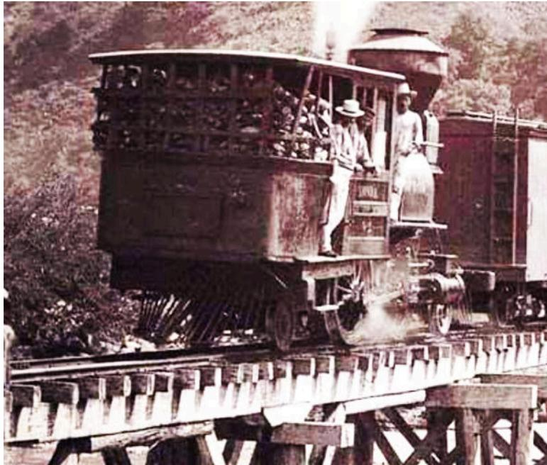
This photo was supposedly taken near Honda and the number and name on the cabside are **2 'HONDA'**. The loco is clearly a 2-4-2ST. The word on the tankside would appear to be 'DORADA' though the initial D is not visible.
