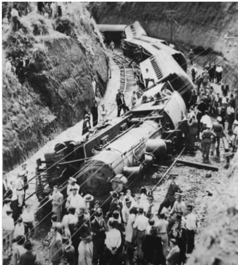
On October 23<sup>rd</sup> 1945 there was a serious accident at Quindio near Armenia on the *FC del Pacífico*. These two images show the aftermath. The loco of the passenger train seems to have been a 4-8-0, and in the photo below it can be seen that it has blind tyres on the second pair of drivers rather than the first. A train from Armenia to Pereira, with locomotive no. **66**, derailed at km 362 two kilometers from Armenia station.
