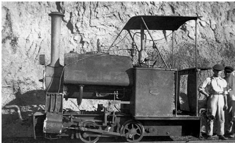
Photo from PCD collection via source [8]. It would appear that an additional cab roof support has been added, rising from the rear of the dome cover, which itself appears to be missing.
