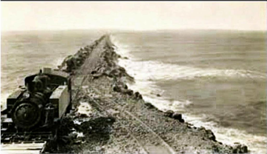
No. 7 out along the big training wall, above, and another of the Porter locos, below, with replacement welded tanks without the original slope at the front end.
