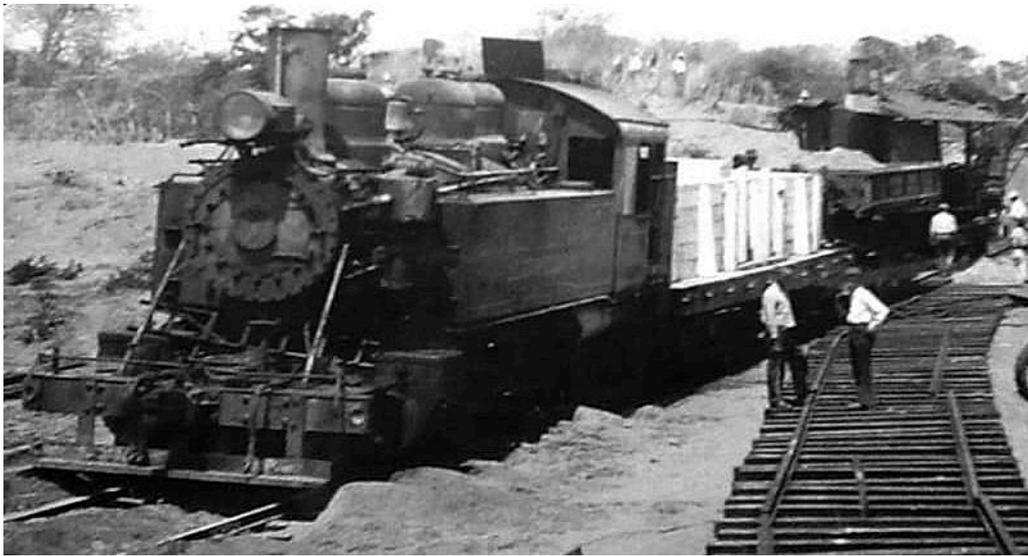
One of the Baldwin 2-8-2Ts in service with a steam excavator. Note that the Baldwins can easily be distinguished from the later Porter engines by their bracing bars from smokebox to buffer beam, and by having their bells behind the front sand dome rather than in front.
