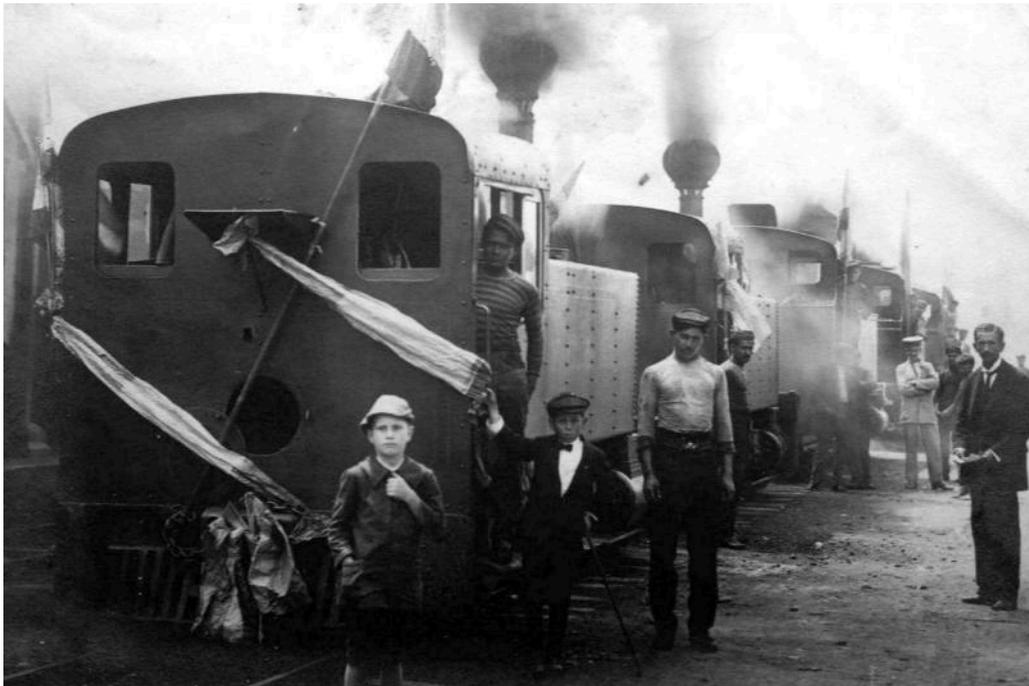
A line of FC de Amagá tank locos raising steam, seemingly for some special occasion. The nearest two are 0-6-0Ts whilst the following three are 2-6-2Ts.
