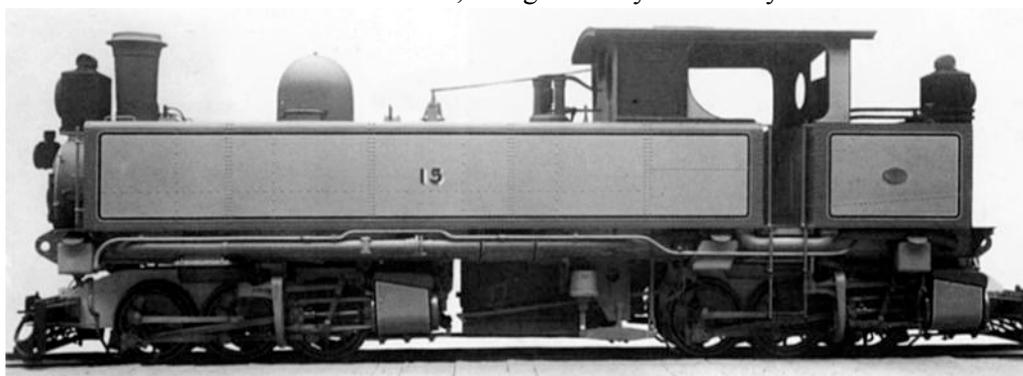
No. **15** is seen in this Kitson works photo to be slightly different from the 1909 pair. [8] The main boiler cradle has lifting eyes at its extreme ends, and there seems to be no rear chimney. Additionally the air reservoirs alongside the firebox on the earlier engines have disappeared.
