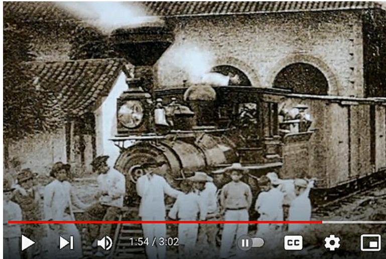
A still from a video showing what looks like a Porter tender engine clearly with the number **9** on the smokebox door. The steam dome is of the later pattern but the sand-dome is an early one.
