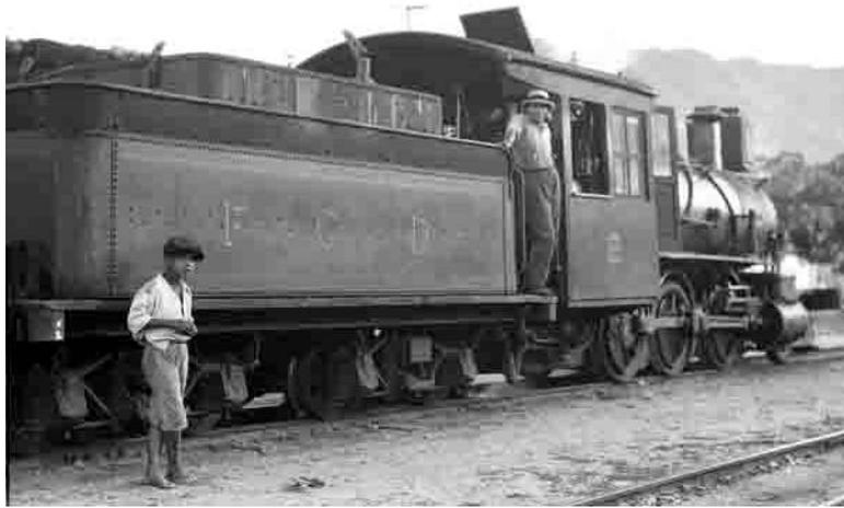
FC de La Dorada no. **2** originally no. **7**. High res versions of this image are available from the Restoration & Archiving Trust via their website; their ref. cijwsam034. The lower cab panel appears to have been encased in steel and the upper cabside rebuilt, whilst the tender now carries an oil tank.
