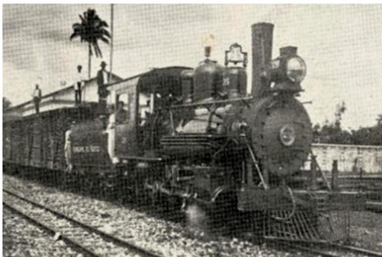
One of the later locos of this class, **24, 25** or **26**, leaving Palmyra for Cali. The dome looks slightly narrower than on the earlier locos, but the distinctive sand-dome topped by the bell is still apparent.
