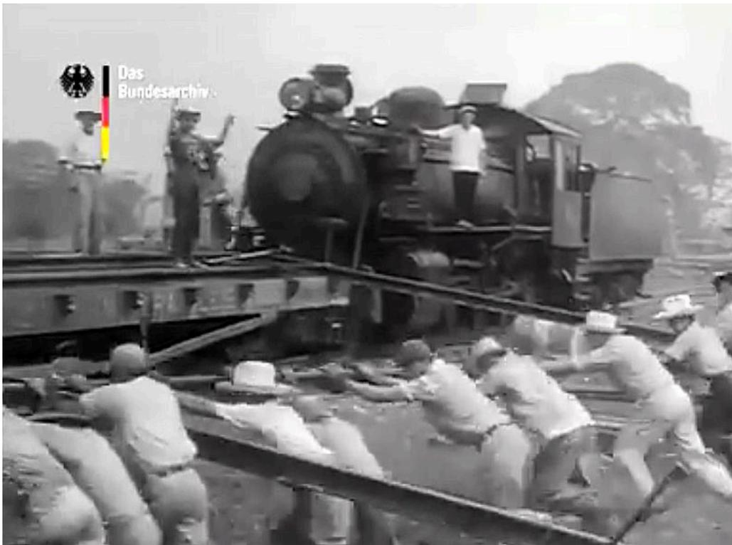
A still from a German video showing HSP 2-6-2 no. **11** on construction trains near Barrancabermeja in 1958. Closer views clearly showed the front number plate, the compound air pump and the lack of sand-boxes protruding above the running plate.
