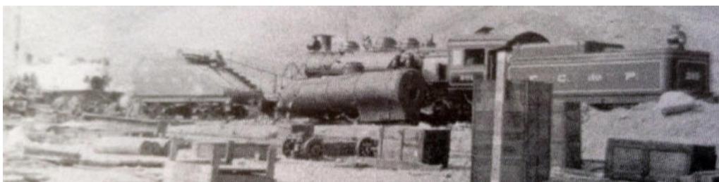
On the left of this photo is again seen an ex-tank loco with the slope-back tender, either in course of rebuilding or when later being scrapped. On the right, behind a dismantled boiler, is the Mallet no. 201. The photo was received from Sr. Pablo Moraga.
