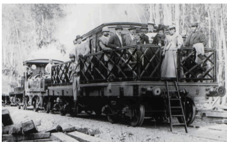
A Manning Wardle 0-4-0ST during Manuel Ossa's contract, on the old bridge in the barrio Guillermo Francke a few hundred metres north of Osorno station. The wagon is an improvised inspection saloon, as is evidenced by the next photo.
