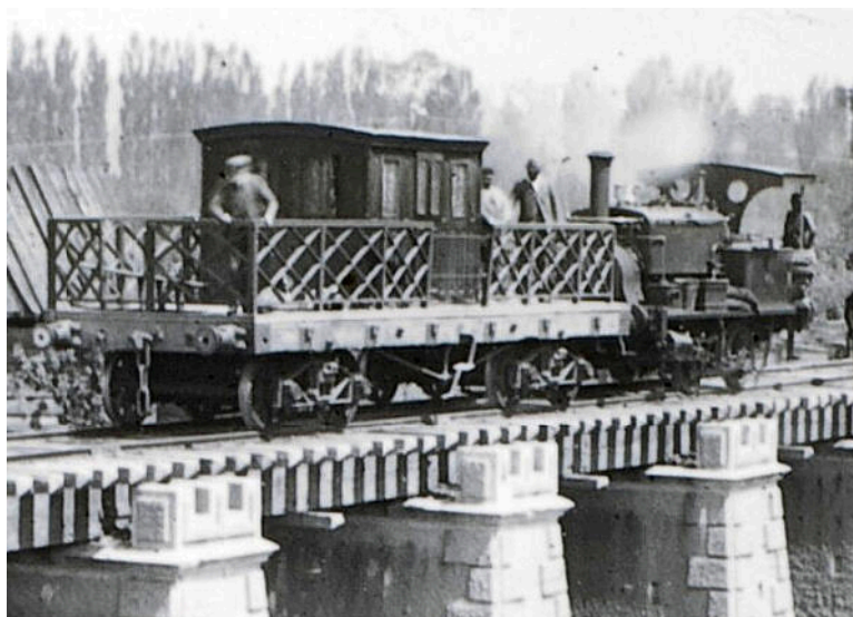
A Manning Wardle 0-4-0ST during Manuel Ossa's contract, on the old bridge in the barrio Guillermo Francke a few hundred metres north of Osorno station. The wagon is an improvised inspection saloon, as is evidenced by the next photo.
