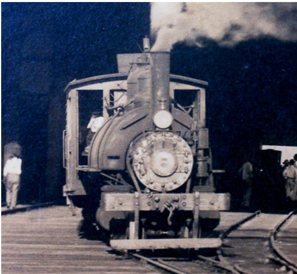
No. 8, rather later in its life and with stove-pipe chimney and shunter's/switcher's steps instead of a pilot, waits beneath the canopy on the jetty at Puerto Varrios.
