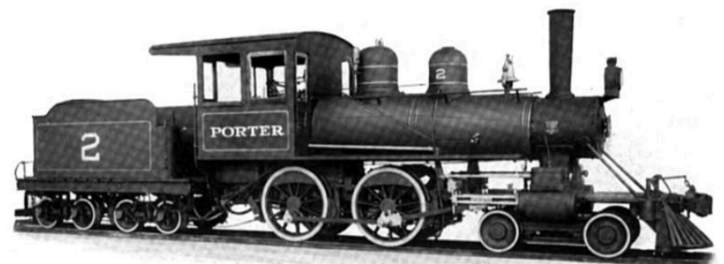
Illustration No. 2, from photograph of 10 x 16 cylinders, 36 inches gauge locomotive, exported to Central America.
