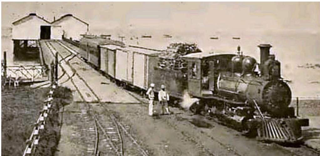
This too looks like one of the SR 4-6-0s, and it has the same modifications noted on no. 10, above. The jetty in the background is that at Acajutla.
