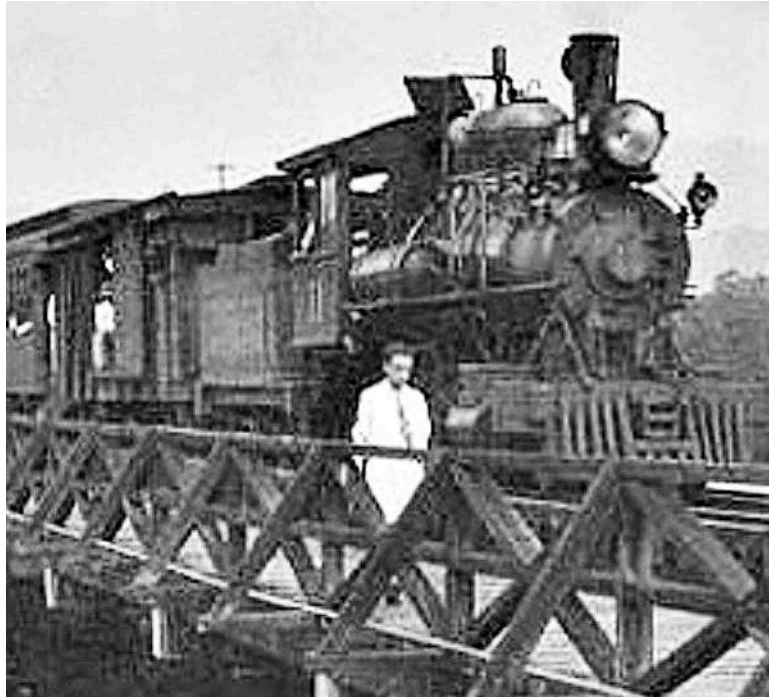
A locomotive no. 11 crosses the lagoon bridge at Puerto Cortes at the head of a passenger train. As with the image of the right side of no. 12 , above, the loco seems to have acquired a strange rectangle of pipes above the dome, possibly a steam take-off line for some purpose.
