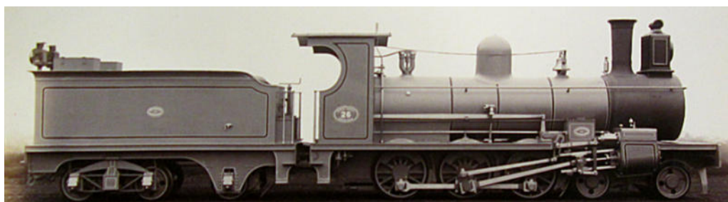
Neilson 4-6-0 no. 26 , as seen in a builders' photo. The 2-4 wheel arrangement
