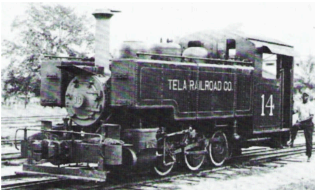
A typical ALCo 0-6-OT produced for Russia but not delivered. Seemingly without change when delivered to Honduras apart from regauging to 3' 6".
