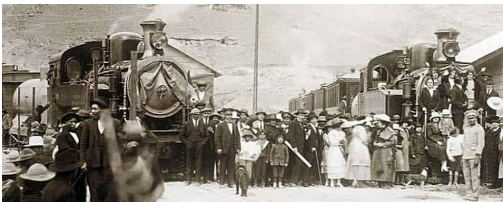
Two Mallets at the head of trains, and seemingly some kind of celebration. Note also the water cart tenders behind each engine. NB It is possible that these were the similar FC Potosi - Sucre - Tarabuco locos, though the double line of writing on the tank-side of the left-hand engine looks very like that shown in the previous photos above.
